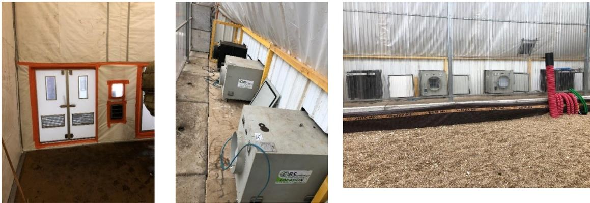
FIGURE 7 : BATIMENT DE DEMANTELEMENT – CONFINEMENT ET SYSTEME D'EXTRACTION D'AIR AVEC FILTRE TRES HAUTE PERFORMANCE
