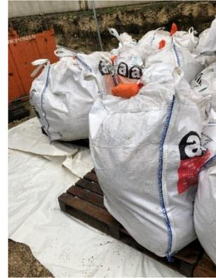
FIGURE 9 : CONDITIONNEMENT DES DECHETS AMIANTES
